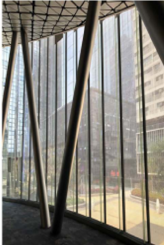
Unpowered rear view picture
